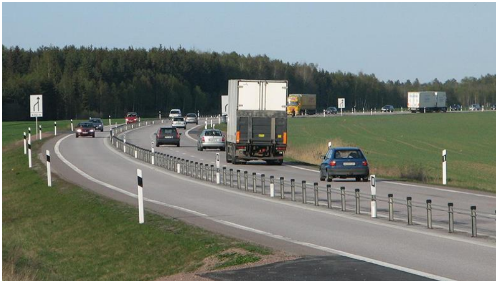
A safety fence known as the “Swedish 2+1 with wire rope median” in Sweden. [Photo: Joel Torsson]
